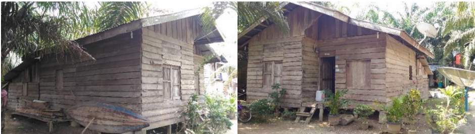
Figure 3 Condition of the Bonai Tribe's House
